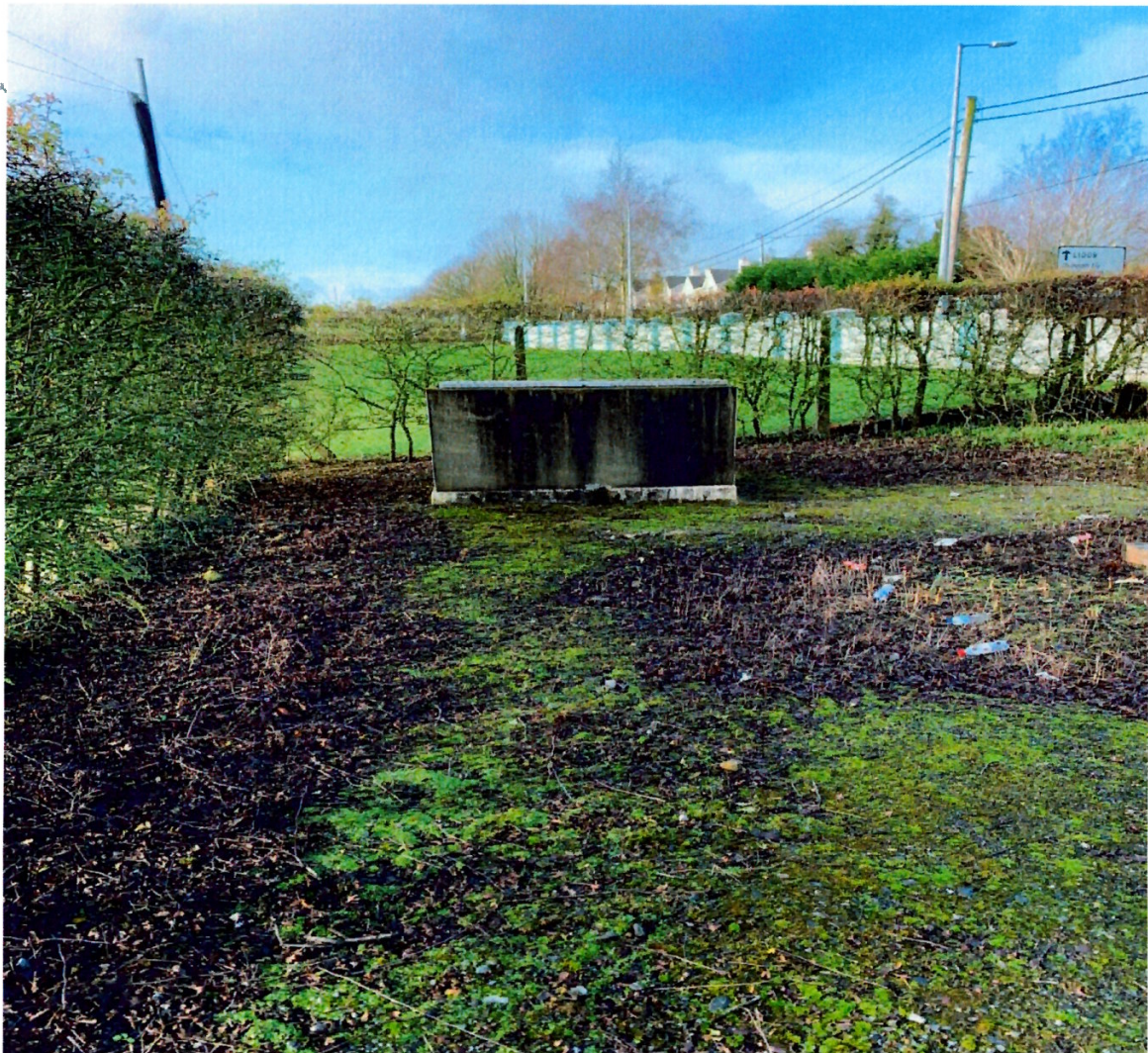
Figure 2.1 – Ballycallan GWS Water Abstraction Compound
